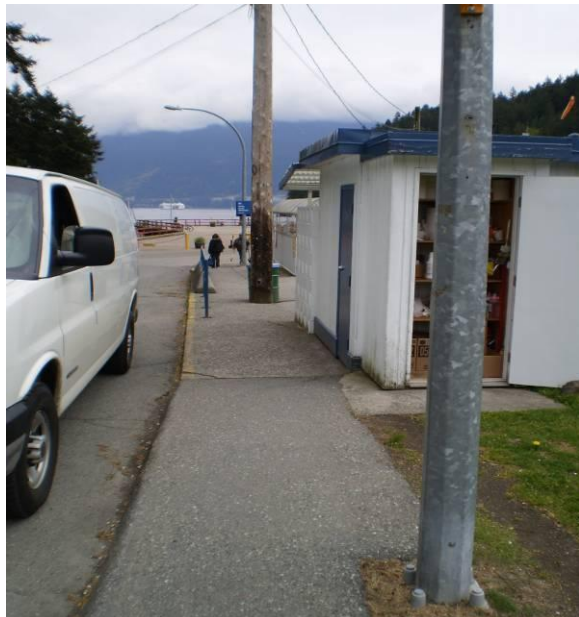
Narrow, uneven pathway, not accessible to scooter or wheelchair
