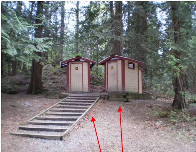
Killarney Lake washroom, located on knoll with stairs
